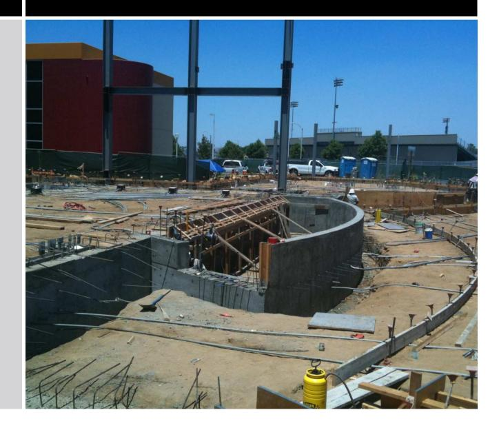
July 7<sup>th</sup>, 2011: Curb forms are being constructed along one of the two ramps leading down to the stage.
