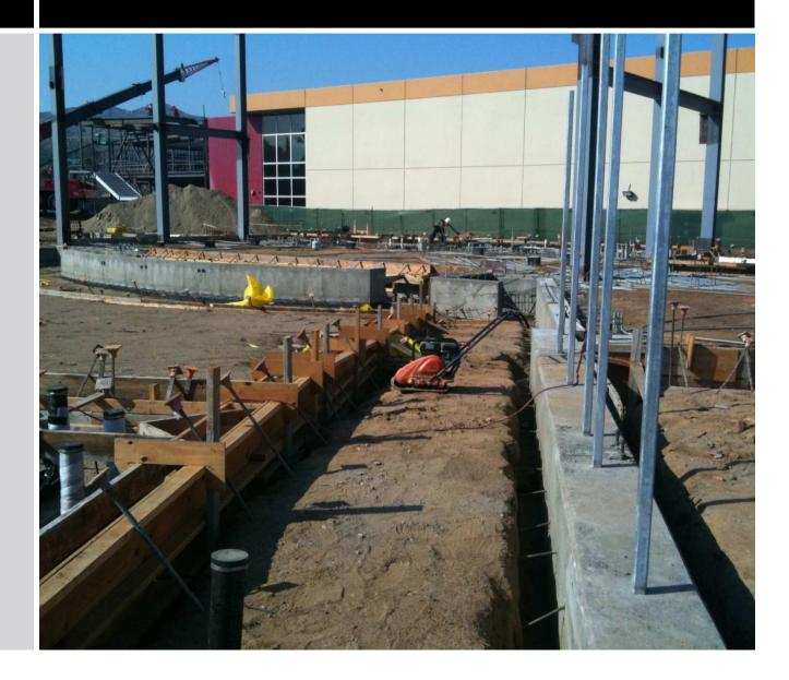
July 14<sup>th</sup>: The seating area slab on grade has been poured and is being finished. In the background the crew is beginning the SOG pour at the stage.
