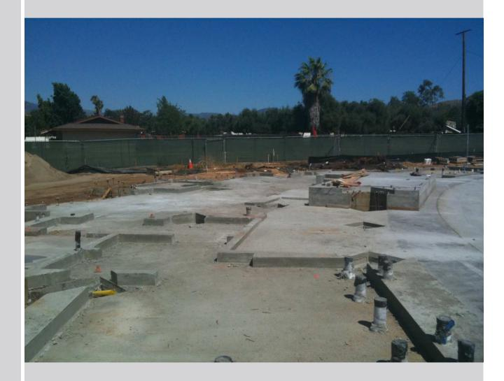
July 21<sup>st</sup>, 2011: The structural steel knife plates are being installed where cross braced frames are required. The columns will be lowered into position over the knife plates and welded into place.
