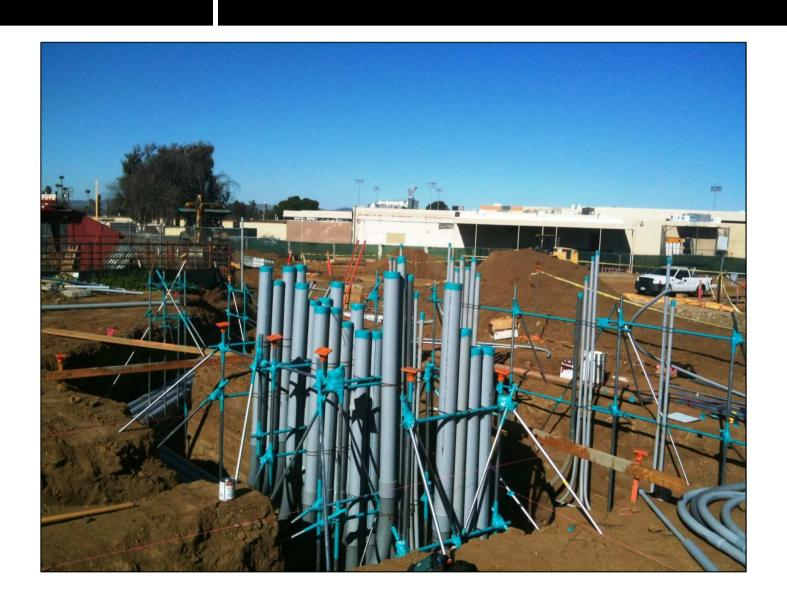
Edison electrical vault and transformer pad are in place and awaiting flatwork to secure in place.
