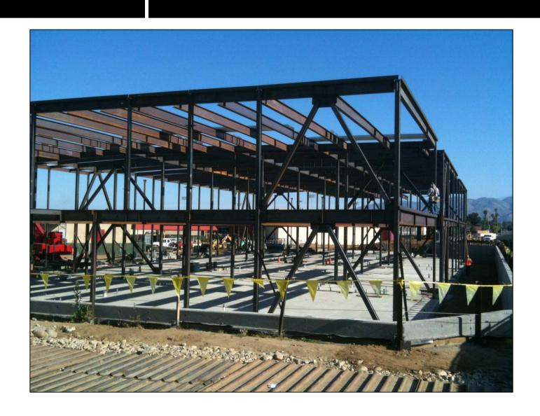
5/5/11: 2<sup>nd</sup> floor deck has been spread and is in the process of being attached to the beams.
