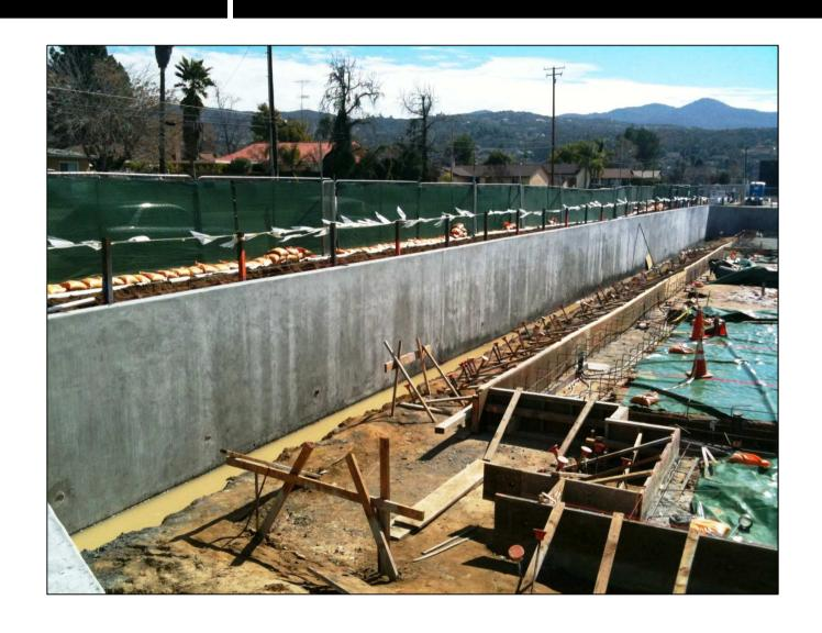
1/26/11: Completed column embeds and grade beams in background. Elevator pit and the elect. data and bathroom footings in progress 2/2/2011
