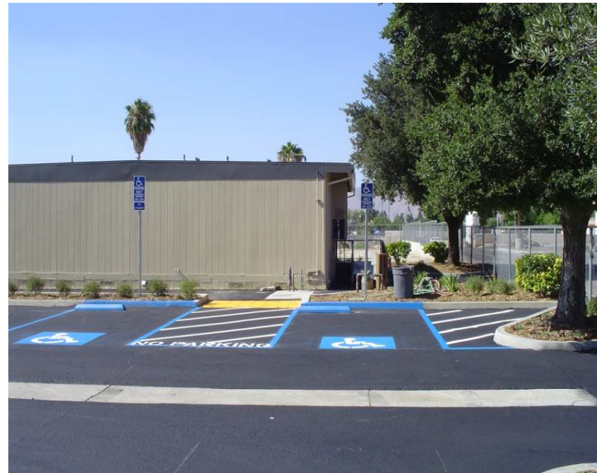
New parking lot striping adding handicap parking
