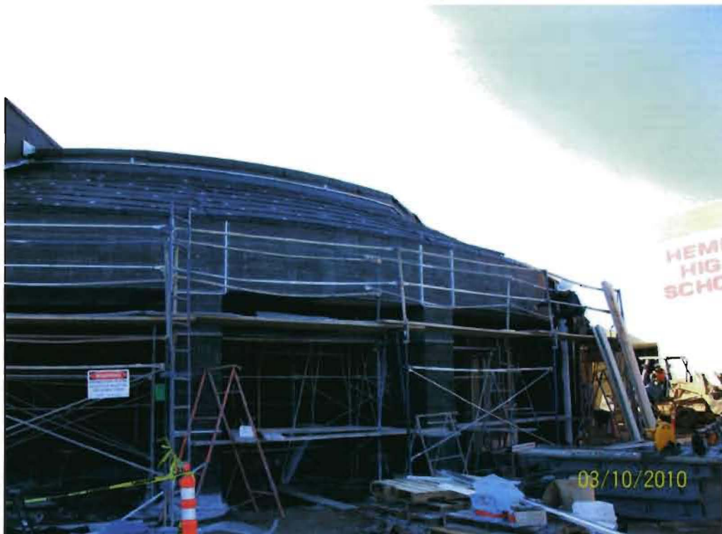
Hemet High School Modernization—Phase 1A New Administration Building—ready for stucco
