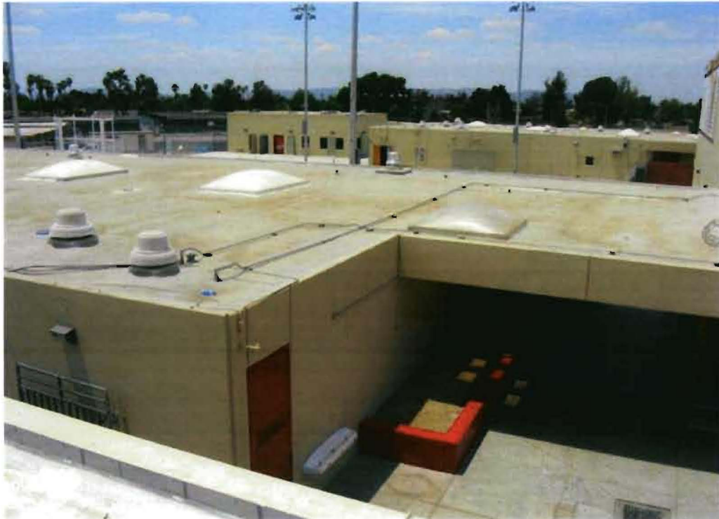
Hemet High School Modernization—Phase 1A Before and After—New Roof and Skylights Girls Locker Room
