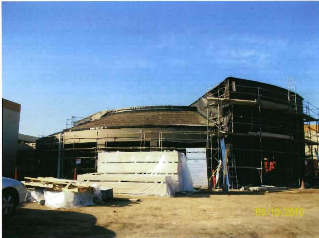
Hemet High School Modernization—Phase 1A New Administration Building—ready for stucco
