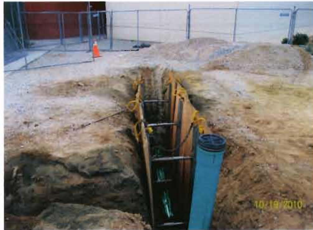
Hemet High Phase 2 – The sanitary sewer at future Theatre Building “A” is nearing completion
