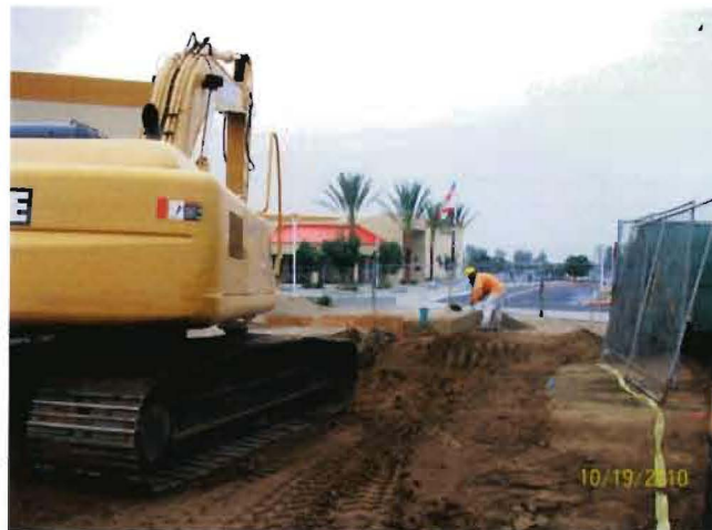
Backfilling sanitary sewer at building “A”
